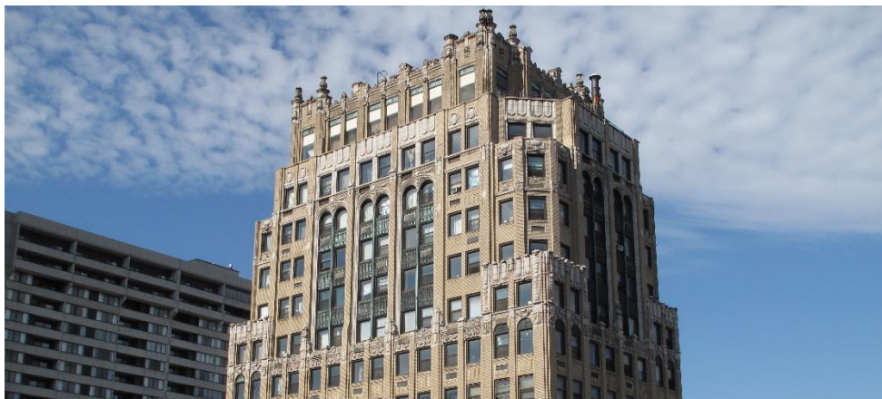
Kemper Stevens Building
