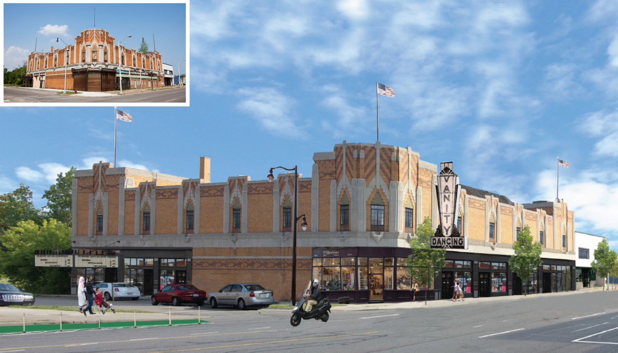
EXISTING AND PROPOSED OF THE VANITY BALLROOM - SOURCE: JEFFERSON EAST INC. (JEI)
