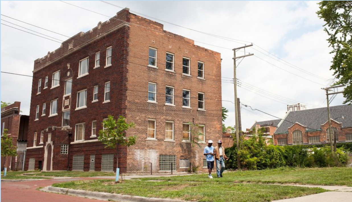
AFFORDABLE UNITS AT IDAO BUILDING (CURRENTLY UNDER CONSTRUCTION)
