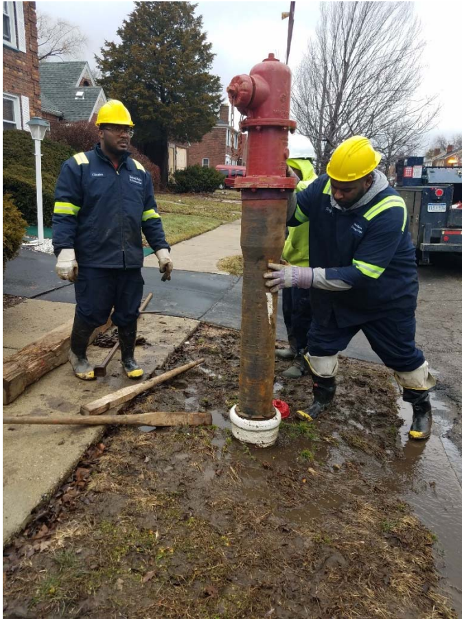
DWSD Field crews installing new fire hydrants
