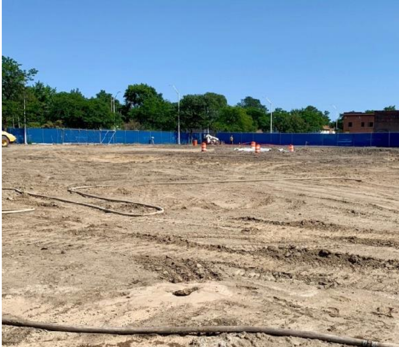
Demolished site of former Brass Factory
