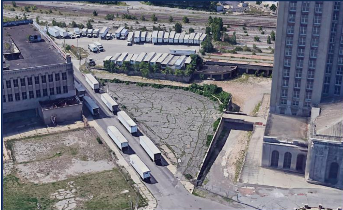
EXISTING NORTH FRONTAGE SITE
