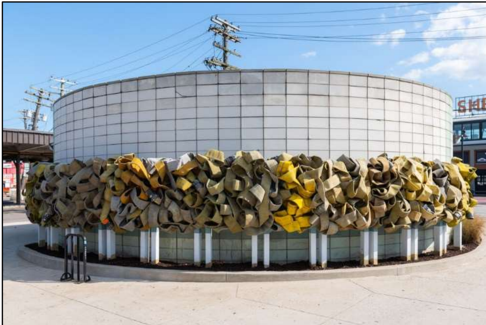
(D) Roundhouse (restrooms) – northwest façade – looking southeast
