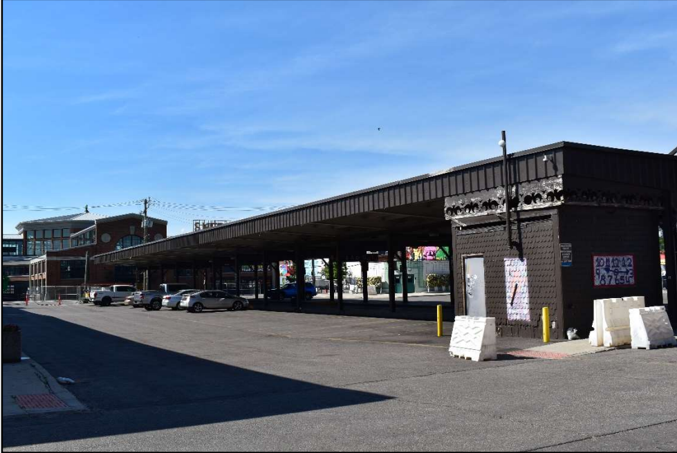
(E) Shed 4 – northeast facades – looking southwest
