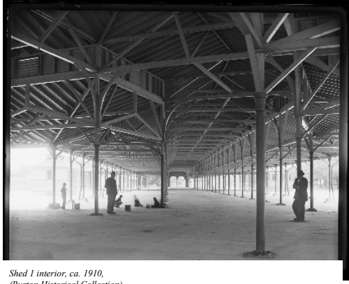
Shed 1 interior, ca. 1910. (Burton Historical Collection)
