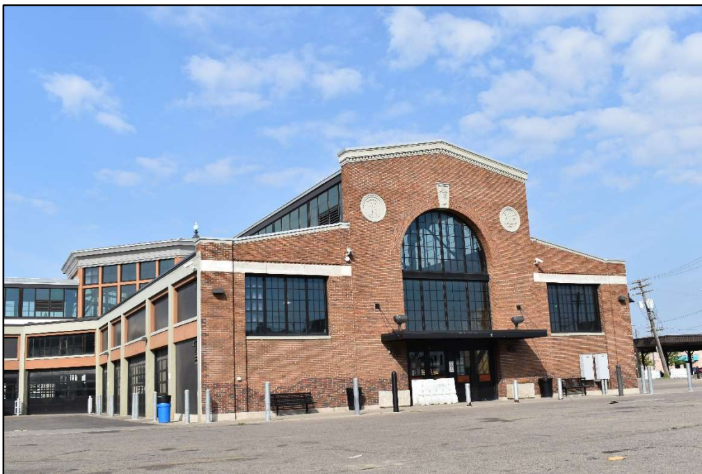
(B) Shed 3 – south façade – looking northeast.
