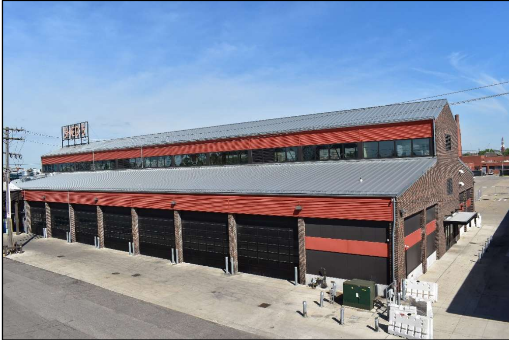
(G) Shed 5 – south and east facades – looking northwest
