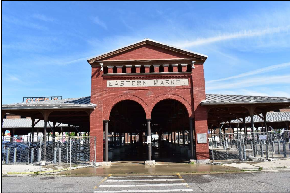
(A) Shed 2 – south façade - looking north
