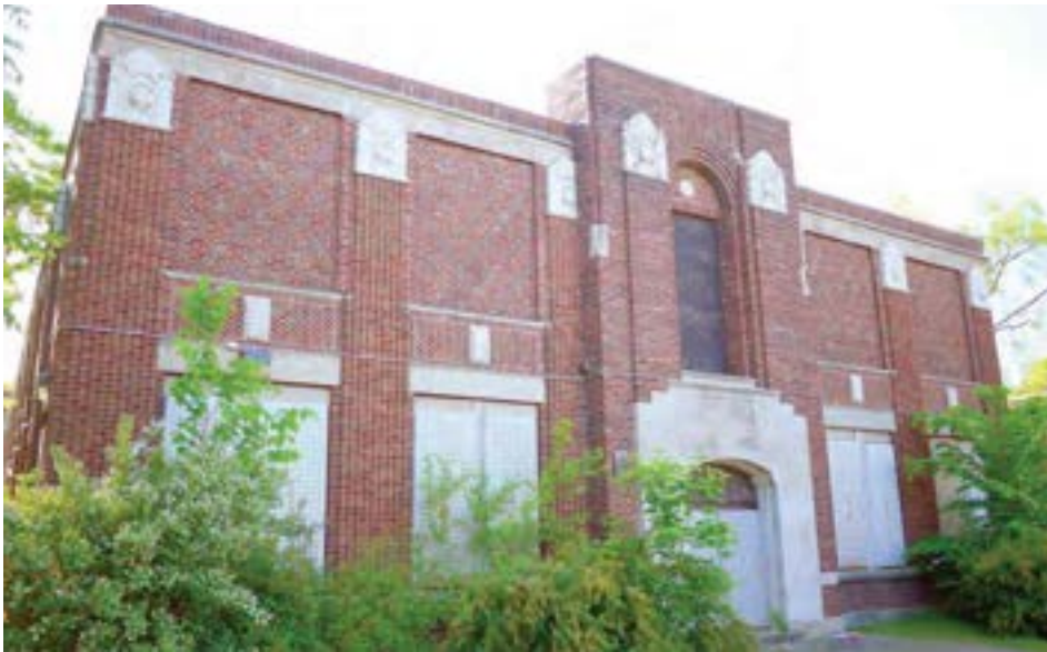
The west elevation of the original 1931 unit, featuring decorative brickwork and limestone and terra cotta embellishments, in an art deco style.
