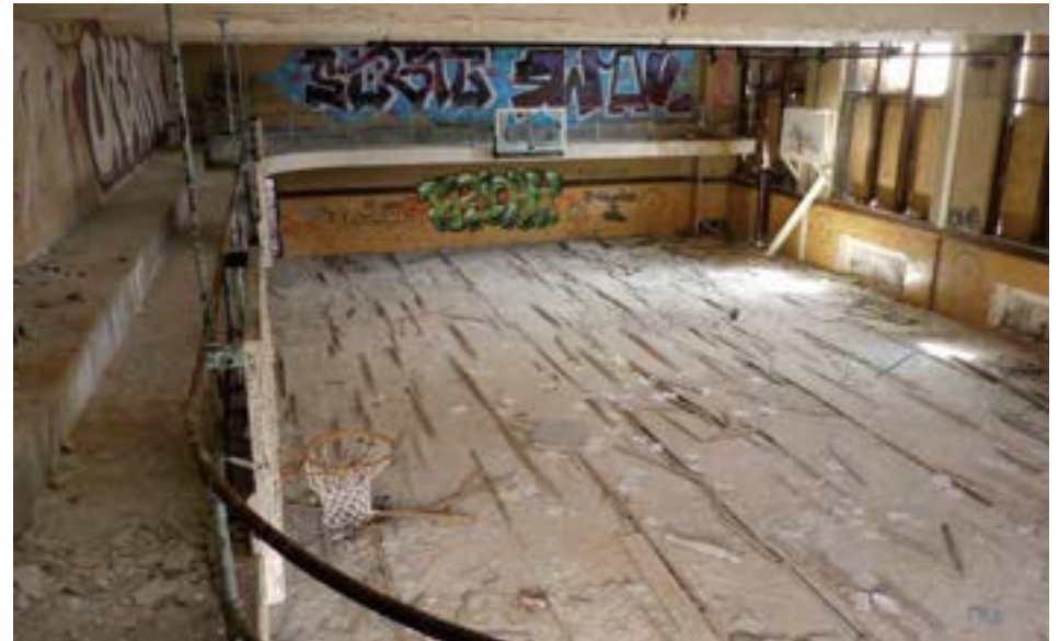
This school has two adjoining full-sized gymnasiums, one for boys and one for girls, each with a mezzanine bleacher area wrapping three sides of the basketball court. Each gym is attached to a large locker room.
