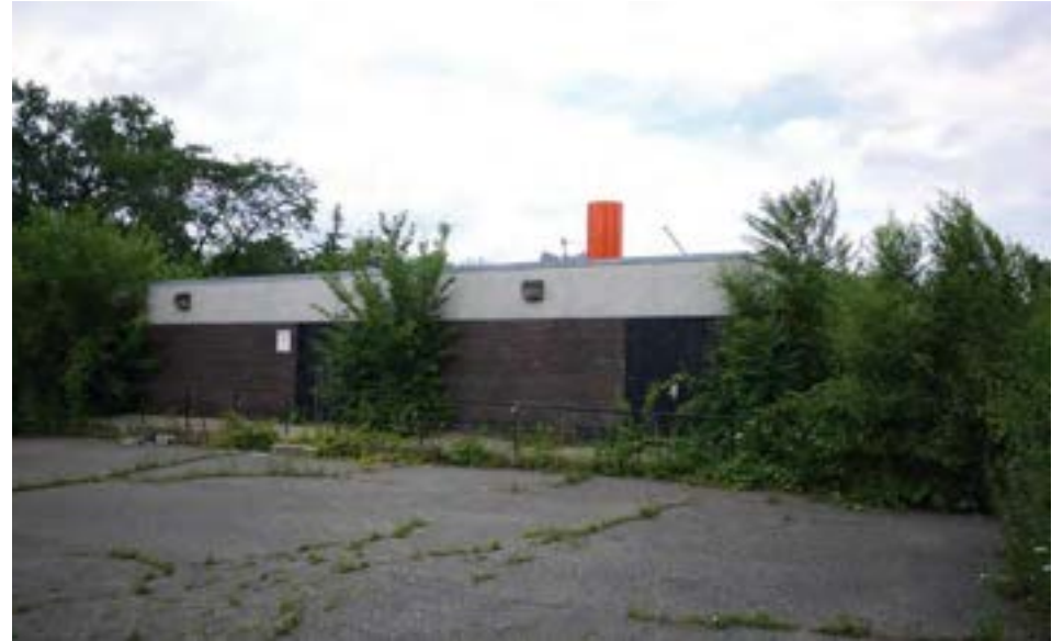
South elevation, from south parking lot. South end of school includes the boiler room and receiving areas. The bright orange smokestack is a notable feature in an otherwise drab school.
