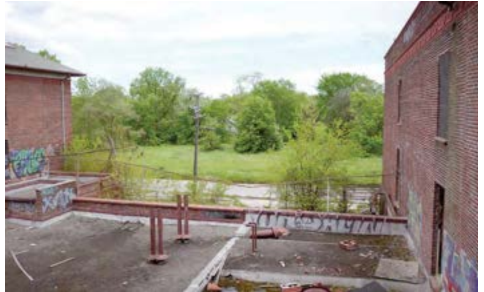
The 1915 and 1919 units created a U-shaped plan with a central space to allow light and ventilation. However, the space is filled by the boiler room roof and is not accessible as a true courtyard. The completely vacant lots that surround the school are visible in the background.
