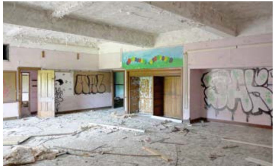
The library is a large space with an open floorplan and ample natural light. The former kindergarten, located directly below, has the same overall dimensions, but was subdivided into offices in recent years.
