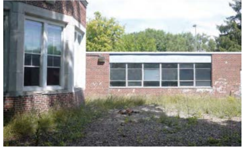
1925 kindergarten bay window at left with 1961 addition behind. Although the 1961 addition uses a modern architecture style and different construction methods, care was taken to match the scale and material palette of the original.
