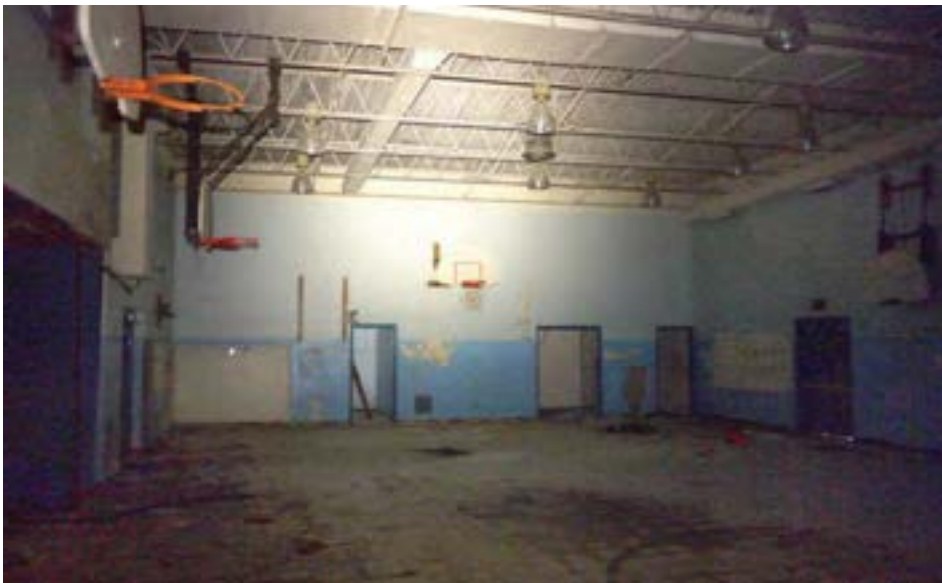
Lynch lacked a gymnasium until the 1975 expansion. The gym is a windowless CMU box with a steel open-web joist roof. The gym is part of a larger L-shaped multipurpose space that also includes a cafeteria and auditorium (pictured above right).
