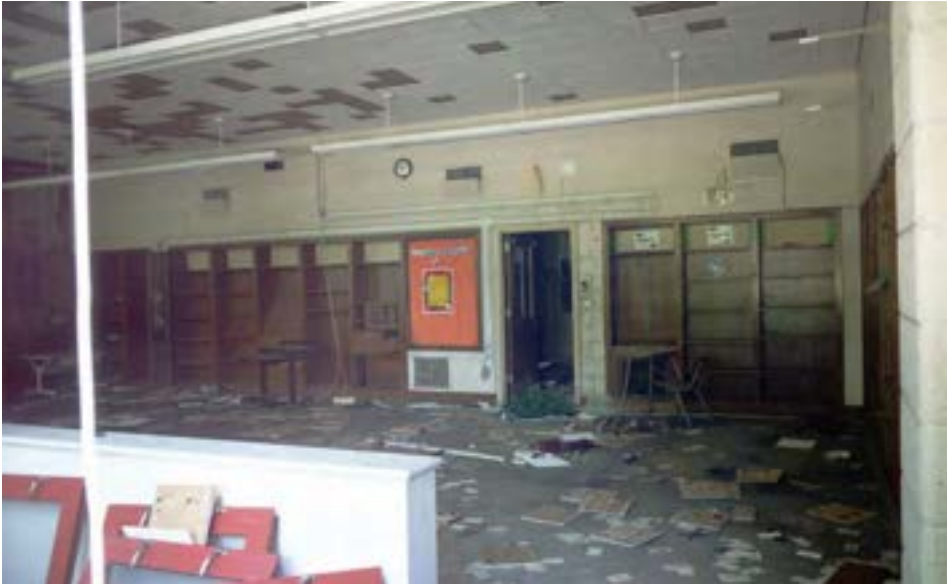
Library (observed from outside)
