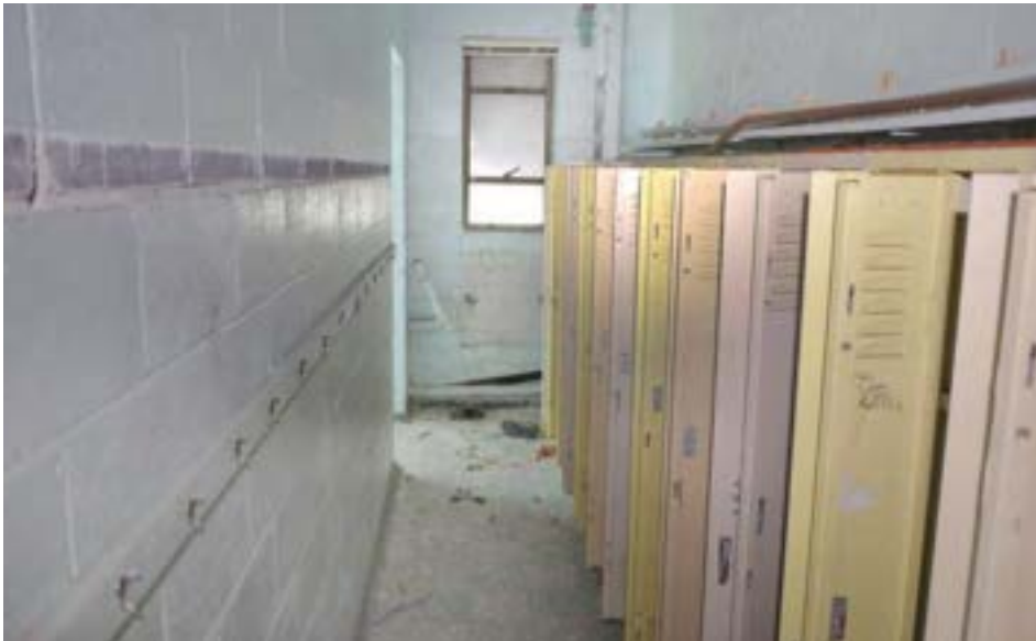
Each of the original classrooms features a walk-in locker/storage area behind the rear wall.
