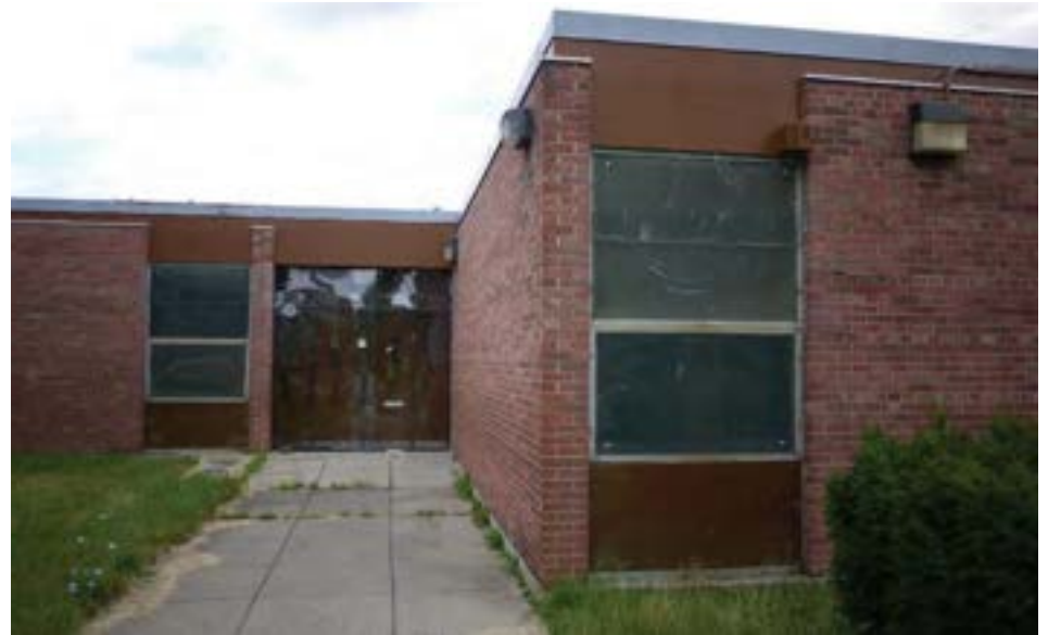
Main entrance located at southeast corner of building (off Ewald Cir). At front right, two larger classroom spaces protrude from the otherwise square footprint of the building.
