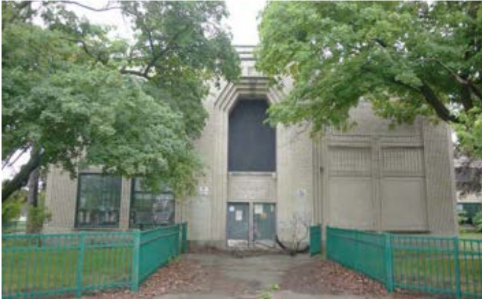
Northeast entrance featuring distinctive art deco-style geometric arch, cast stone school name frieze, and decorative brick work.
