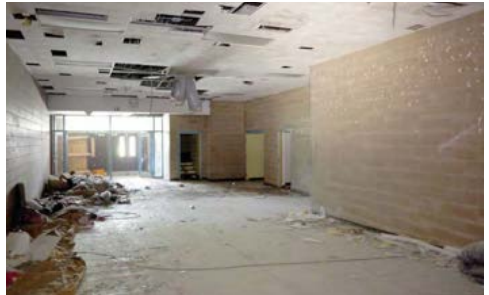
The 1992 unit has hallways up to 20' wide, ideal for accommodating large groups of people attending events in the gym or auditorium/cafeteria. Hallways have no natural light except from the entrances.
