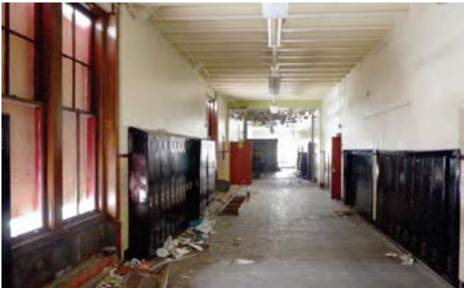
The south corridor is single-loaded, with classrooms facing the street, and windows facing into a central courtyard. Lockers and interior finishes are still in good condition.
