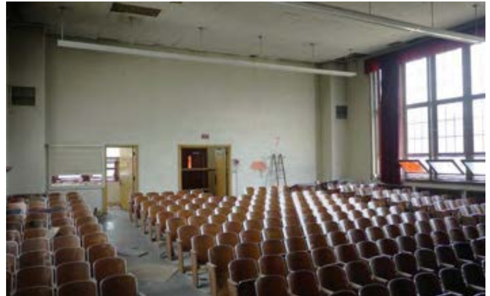
Auditorium with original seating intact. Replacement windows in good condition.
