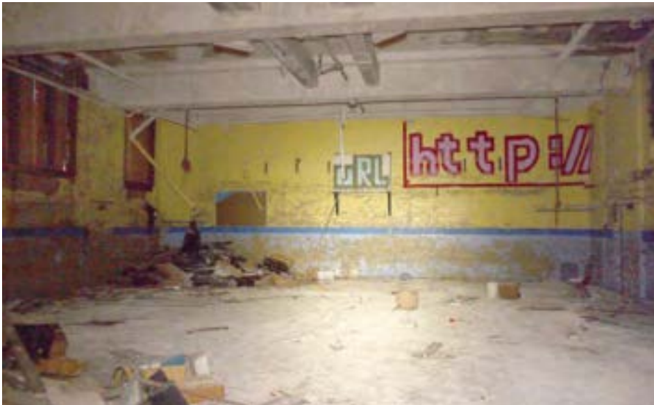
The gym is located in the basement beneath the auditorium. The gym is located several feet lower than the rest of the basement to allow for 18' ceilings. The windows in the left of the frame are located just above grade.
