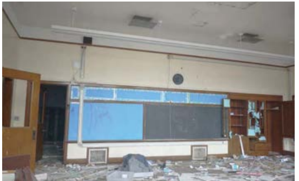
Classroom in 1921 unit, showing plaster walls (observed from outside)
