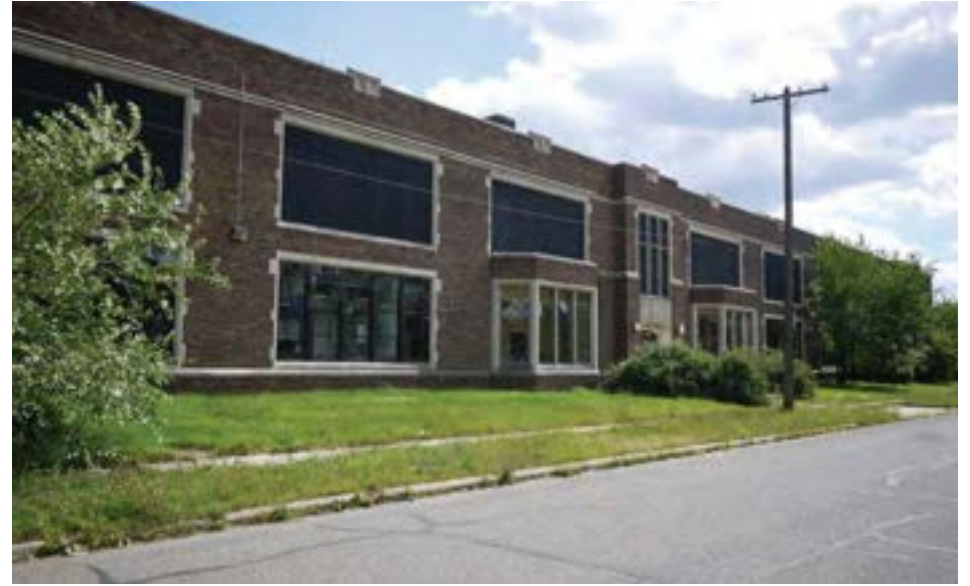
North elevation, with dual kindergarten bay windows visible flanking the side entrance.
