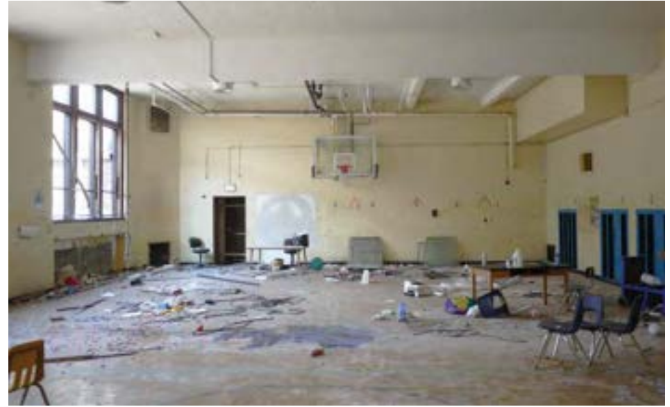
The gym has large, low windows for lots of natural light. The space is in generally good condition, except for vandalism of the floor.
