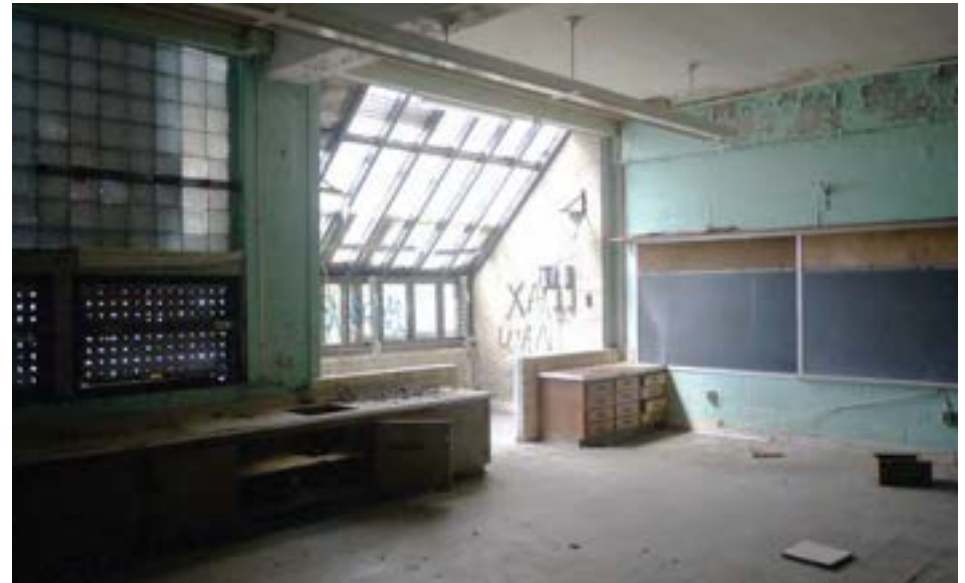
The science room features a south-facing conservatory with a sloping glass roof. This conservatory is more solidly built than those seen at other schools, and feels more directly part of the classroom itself.
