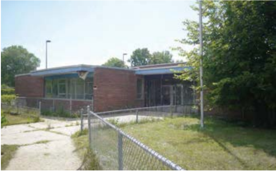
North (main) entrance in 1961 addition. The entrance area is located on a cul-de-sack with a turnaround drop-off area.
