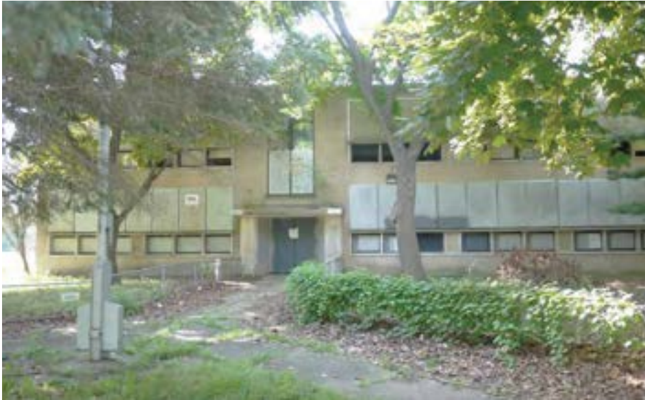
Main north elevation is green and pleasant with mature trees. Steel security panels cover continuous bands of glass block above visible windows.
