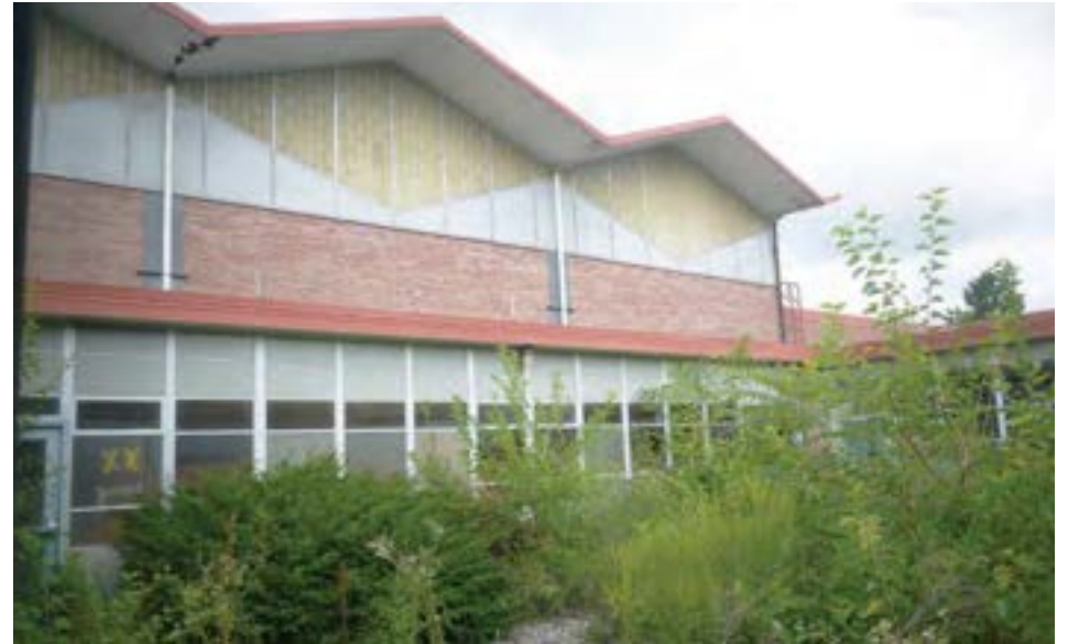
Gymnasium exterior viewed from central courtyard. The gymnasium has a unique folded roof echoing that of the main entrance area.
