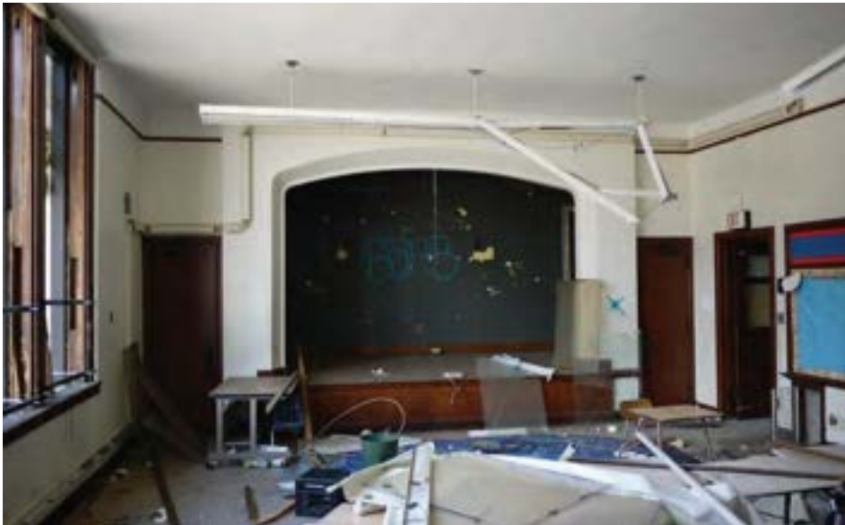
A small secondary auditorium occupies the space of a typical 22x30' classroom, with a miniature stage inside.
