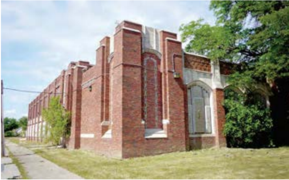
Exterior viewed from southwest corner.
