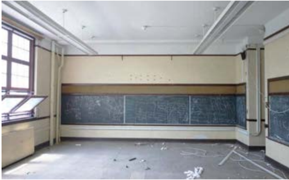
Typical 1921 classroom in good condition, including intact aluminum replacement windows.
