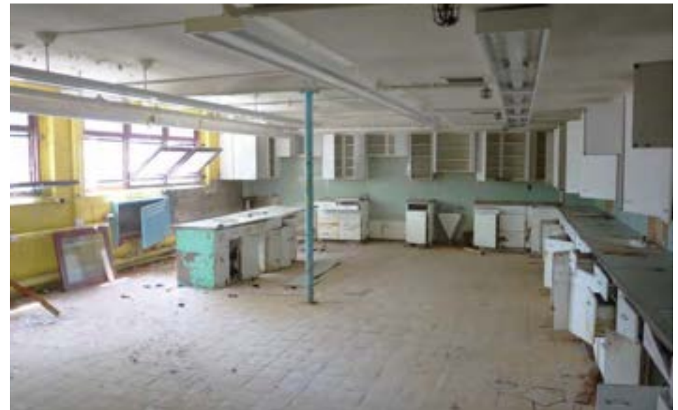
Large cooking classroom in basement of 1921 unit. Cabinetry is intact, but plumbing and fixtures have been taken.
