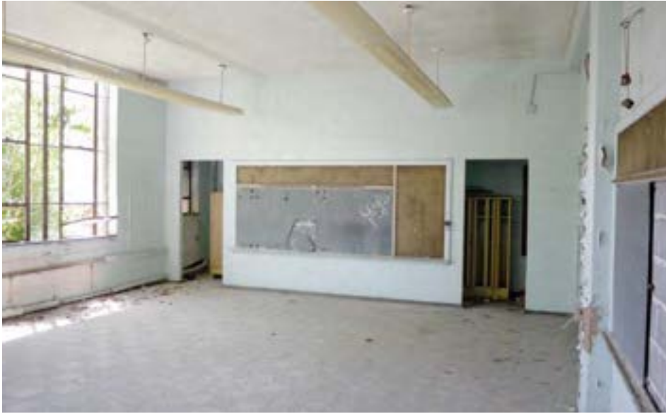
Classrooms in the original unit are simple painted concrete block. There is no built-in furniture like typical DPS-built schools, but classrooms feature walk-in storage/coat areas behind the rear chalkboard wall.
