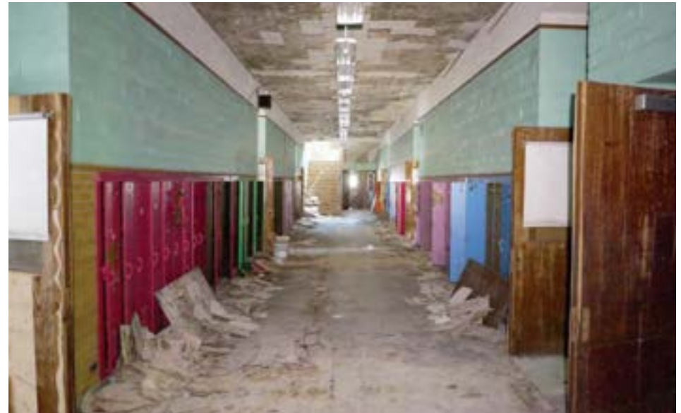
Hallway with CMU and glazed-block walls, and intact lockers.
