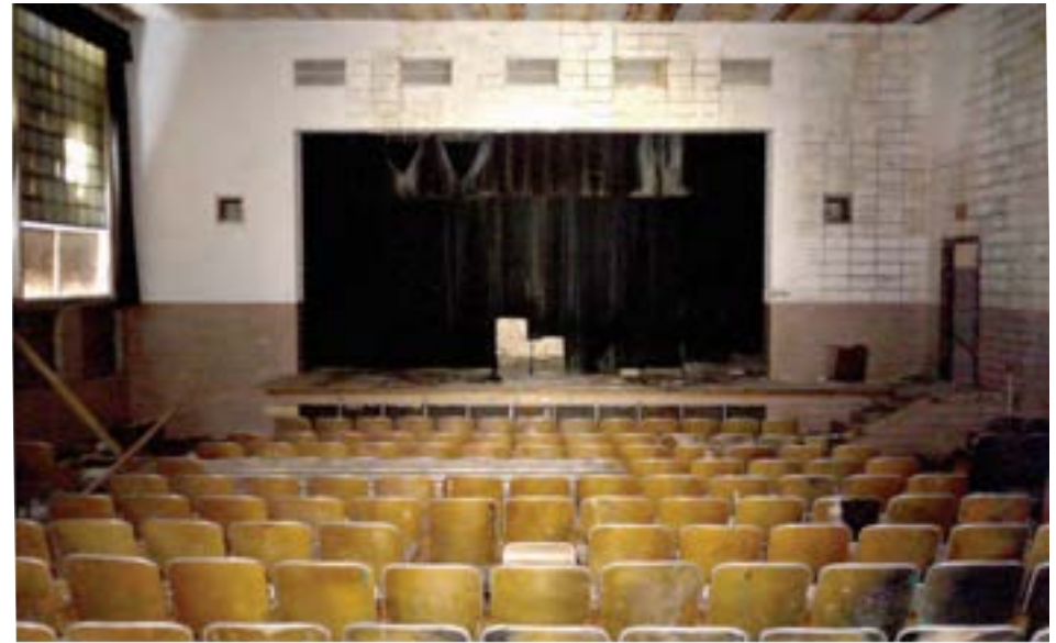
The auditorium is a plain CMU box with large glass block windows.
