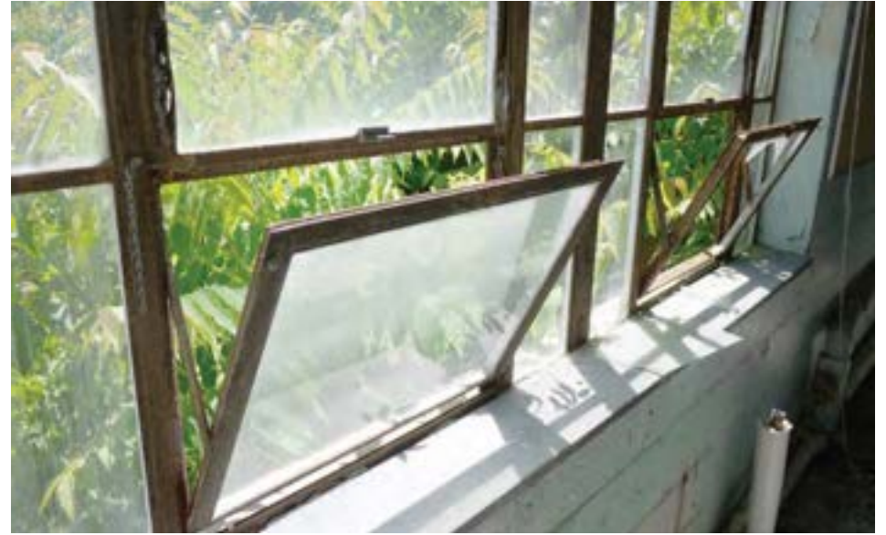
Original steel-frame windows with a large irregular grid are intact throughout.
