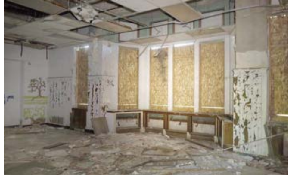
The library consists of two identical, side-by-side rooms, each with a large bay window that faces Dequindre Street. The original 16'4" high ceilings and the tops of the bay windows were concealed by a drop ceiling.
