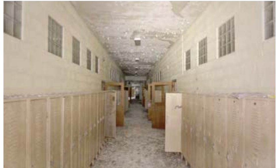
The corridors in the original classroom wings are tall and narrow. Students originally stored their belongings in the classrooms, but banks of freestanding lockers were eventually added to the hall, making it more crowded. Small glass-block windows allow some natural light to filter in from the classrooms.
