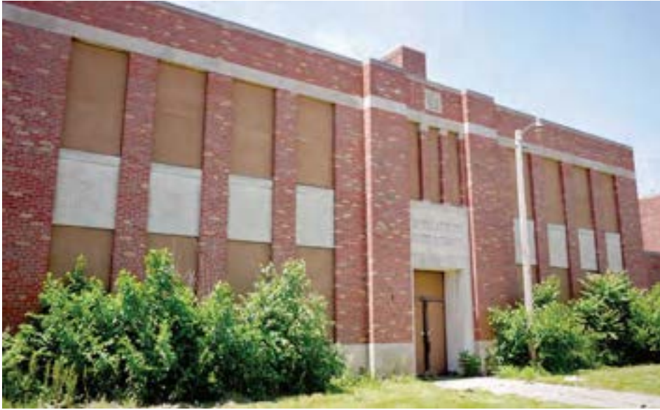
The facade is red brick with geometric cast stone elements in an art deco style. Tall, narrow windows and articulations in the facade emphasize the verticality of the building.
