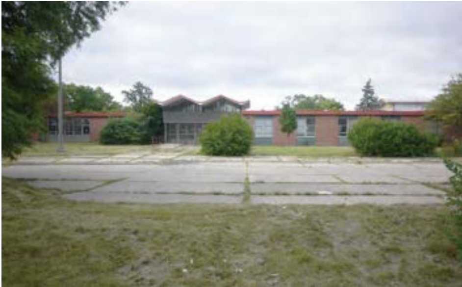
North (main) elevation, showing the folded roof and glass box of the main entrance lobby.
