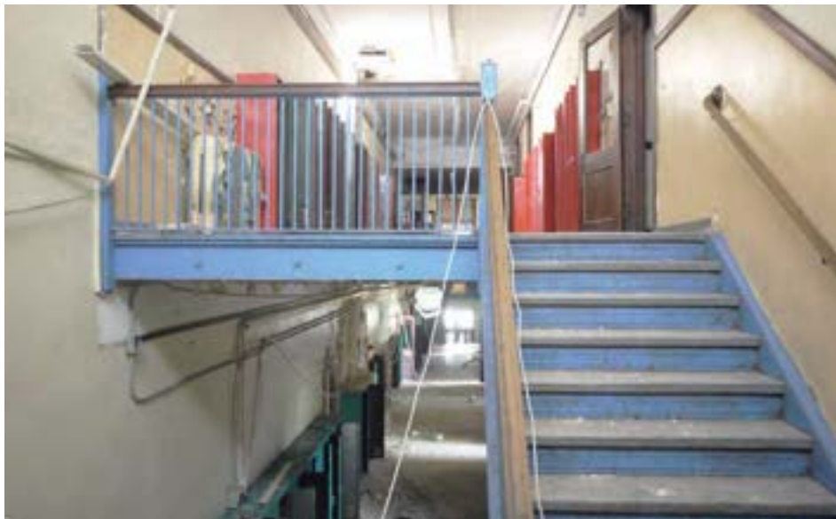
Split-level view at connection between 1921 and 1950 unit. View is from 2nd floor of 1950 unit looking up to 2nd floor and down to 1st floor of 1921 unit. Due to level changes, this school is not handicap accessible.
