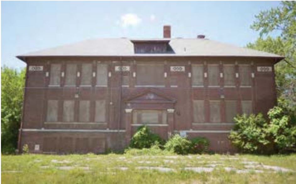
Original 1914 unit east facade (formerly main entrance).
