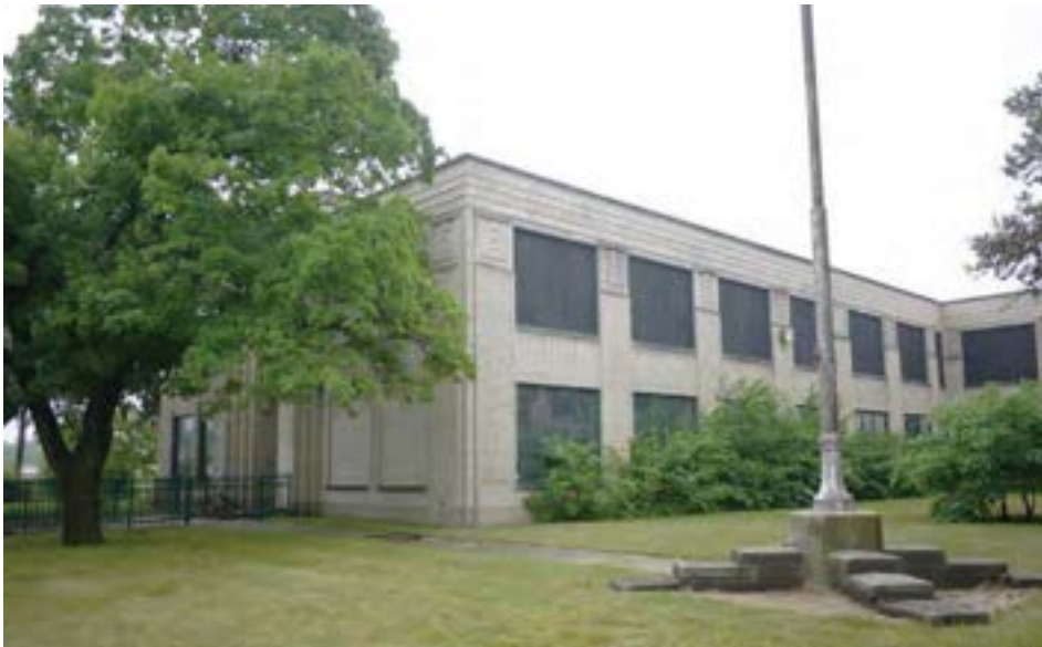
The Northeast wing and front courtyard area. Art deco-style cast stone elements and decorative stack bond bricks are visible between the large square windows.
