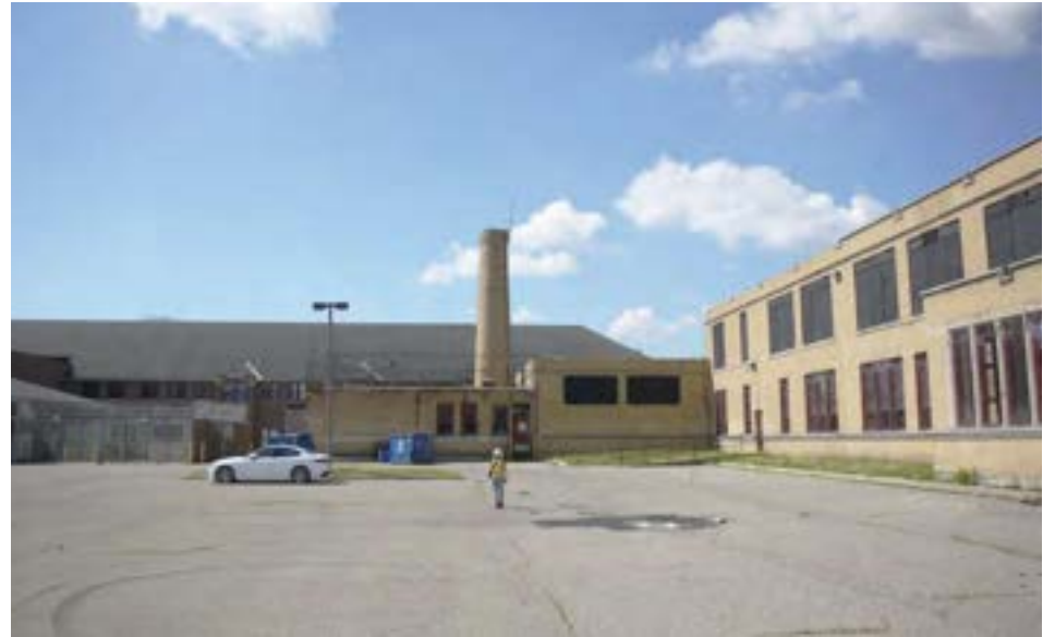
East elevation, showing gym and boiler room, and roofline of new Marion Law Academy school.
