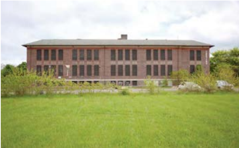
North elevation seen from the large school yard. The right half of this elevation is the original 1915 unit, and the left half is a 1919 addition; expansions were designed to maintain a seamless and unified composition on the primary facades.
