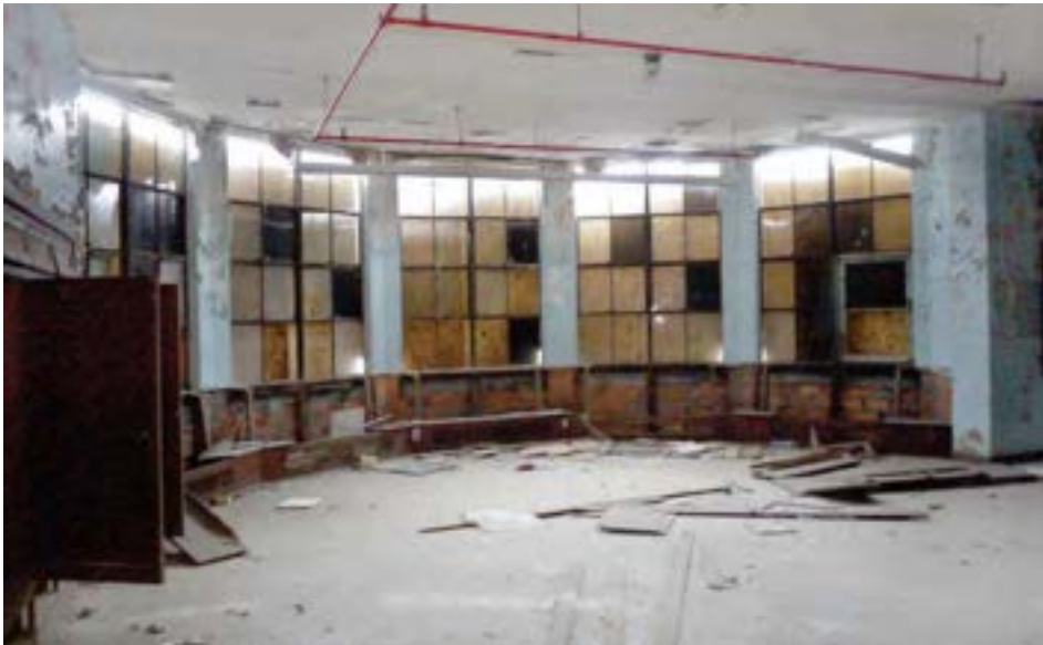
The original 1925 north wing features a kindergarten with a large bay window and a fireplace—a common feature of Detroit schools from this era.
