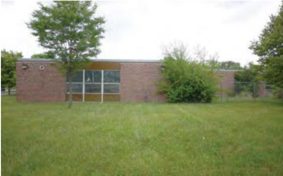
East elevation viewed near intersection of Dexter/Ewald. School is positioned in center of parcel, leaving open green spaces to the east and west. East green space is partly fenced in, but not a particularly safe area for children to play, due to proximity to busy intersection.
