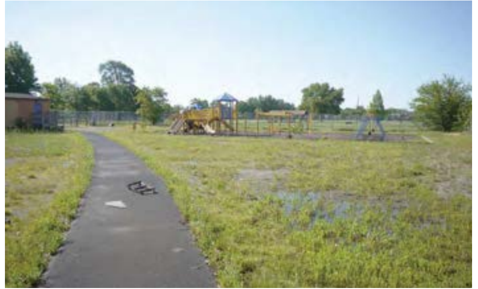
School yard facing south toward Egan Wish Field. Trix playground equipment is in excellent shape. School grounds also include a paved walking path, raised garden beds, two temporary classrooms, and a brick out-building.
