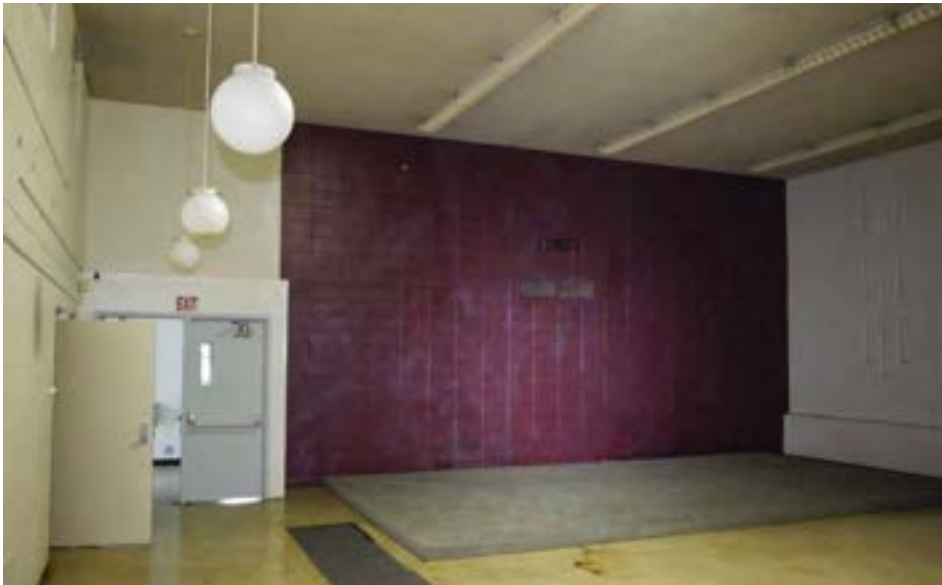
A small gym/multipurpose room is located at the west end of the building. The stage was likely added by the previous tenants, a church. Although windows are covered, natural light can be provided via clerestory windows on the east wall (top left) and glass block slot windows (far right).
