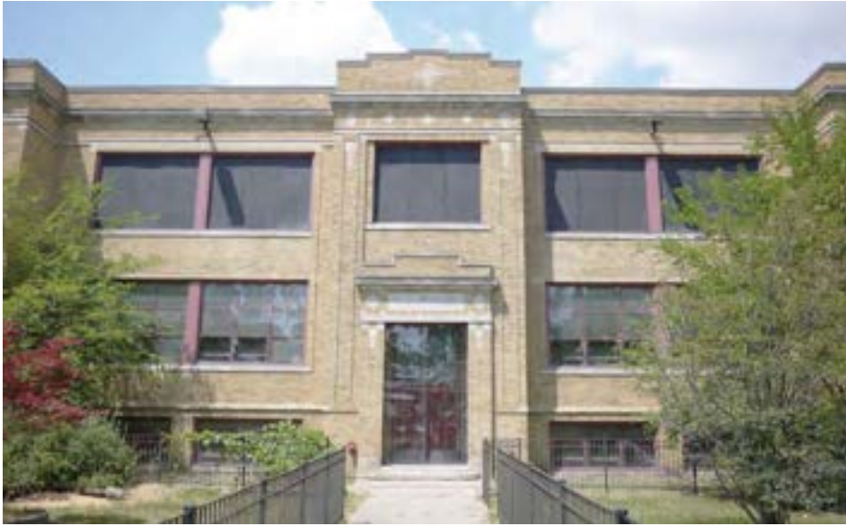
South facade of original 1921 unit, facing Outer Drive
