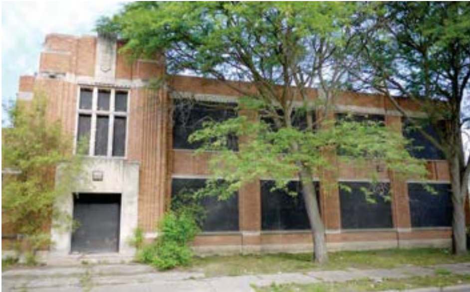
East elevation with vertical brick details and decorative stone details. This wing was constructed as part of the second addition in 1951.
