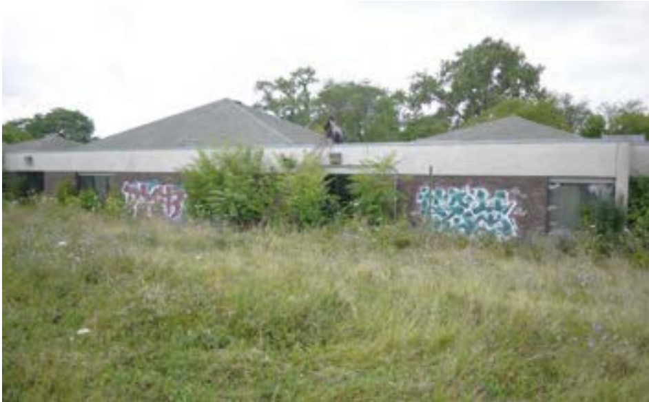
East (rear) elevation viewed from Salsinger Playfield. School has multiple exits leading to park, including from the multipurpose room (gym/cafeteria) visible beneath the larger pyramid roof.
