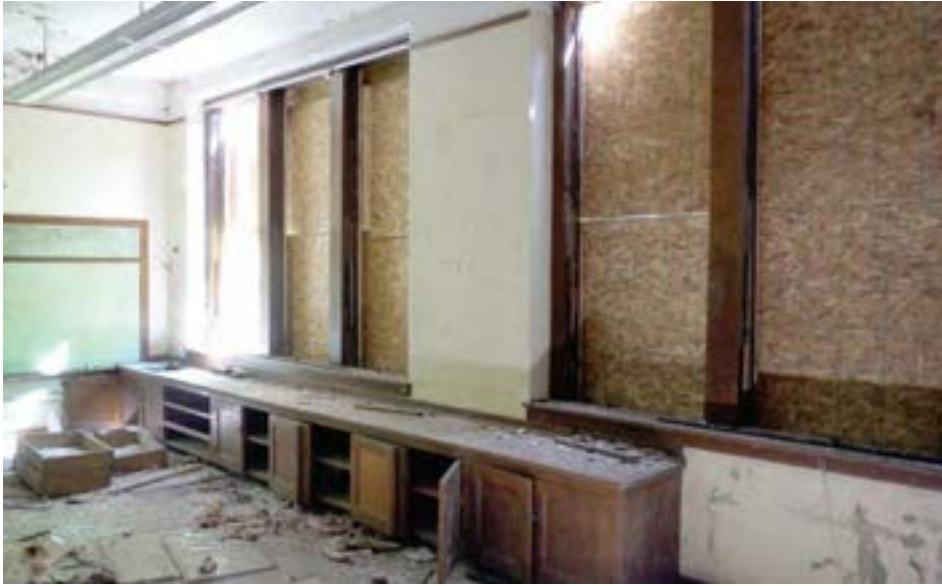
A classroom in the 1931 unit, featuring plaster walls, wood window frames (scrapped), and original wood cupboards beneath the windows.
