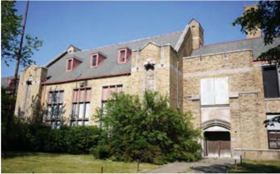
Courville's west elevation is anchored by a central auditorium with high gabled roof. The school features a beautiful gothic-style exterior with decorative brick and stone details throughout.
