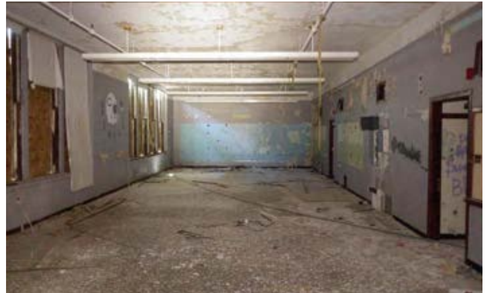
As a former vocational school, Crockett has a number of double-length classroom spaces that were used as workshops and training rooms. On the first floor, many of these large rooms also have extra-thick wood floors, meant to stand up to operating machinery and heavy wear and tear.
