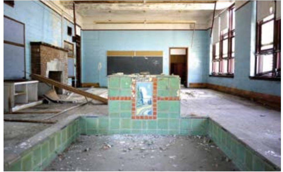
Detail of decorative tile basin in kindergarten.
