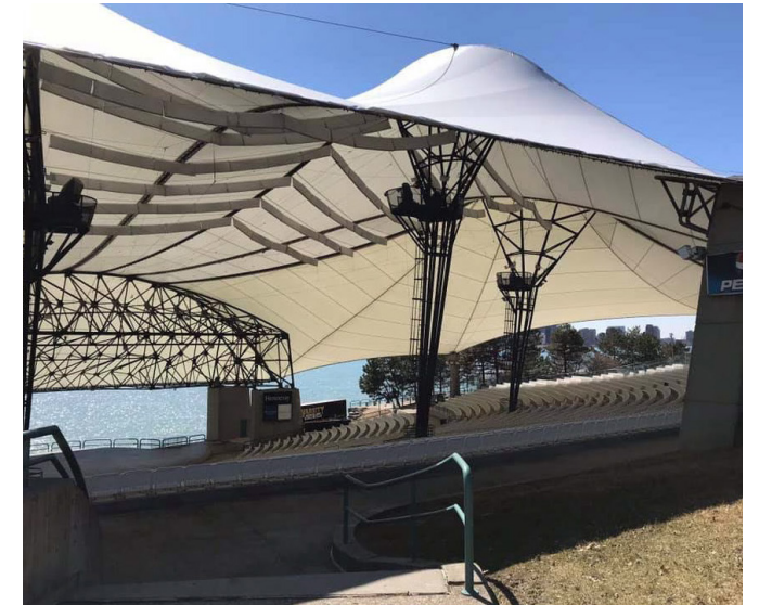
Amphitheater tensile roof over fixed seating
