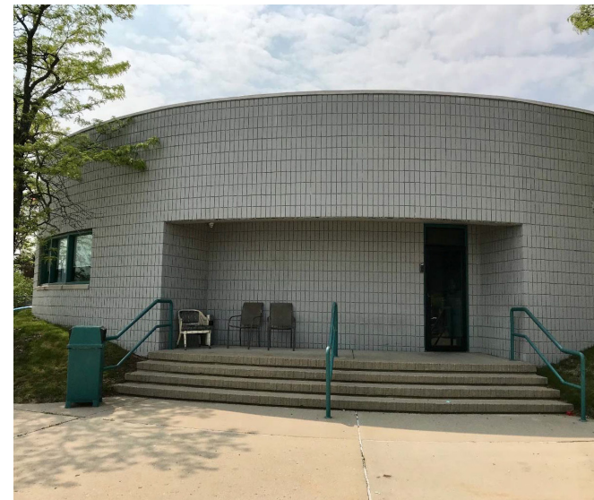
Administrative Office building
