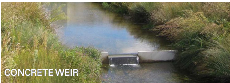
VERTICAL SLOT WEIR
