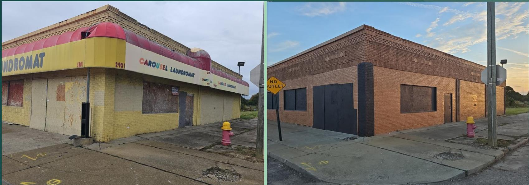
**REMEDATION OF OBSOLETE SIGN/AWNING, PHONE BOX/CONCRETE REPAIR, PEELING PAINT, WEEDS**
