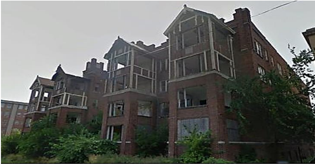
Location 2. 5260 W Chicago Former Structure (Pre-Demo)
