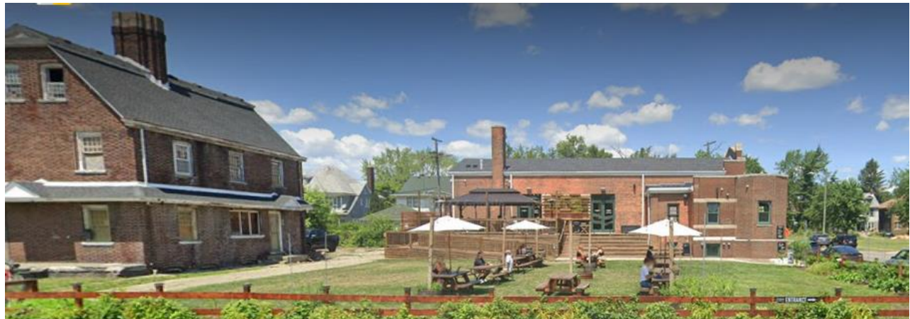
Farmers Market & Rectory under construction future home to Pizzeria
